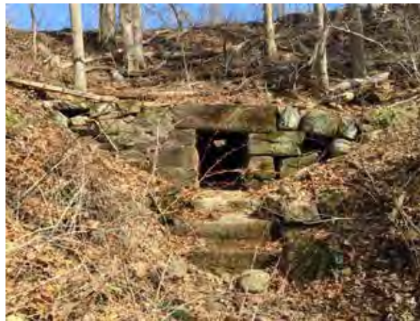
Draining culverts in Portland, CT. Original drainage features can be found throughout the corridor and offer an opportunity for visitors to look back in time and envision the original construction efforts that made this park a reality.
