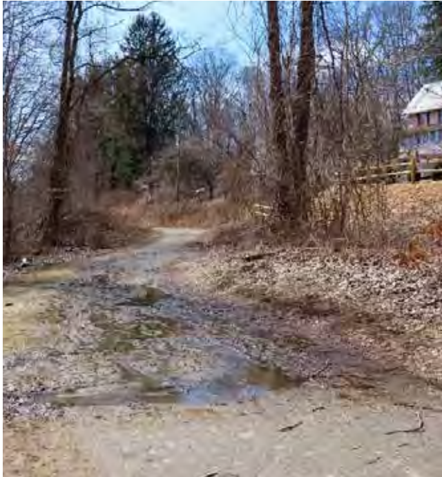
ALSPT Trail surface erosion from rain event
