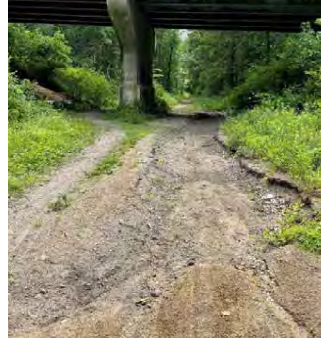
Trail erosion from highway stormwater in Thompson
